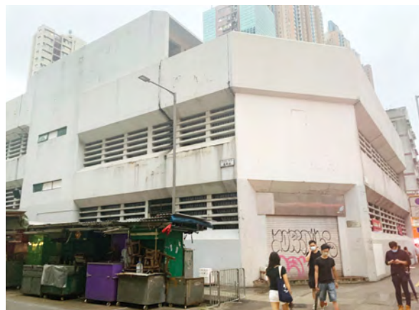
The ex-Mong Kok Market Building will be retrofitted into an interim District Health Centre for completion in early 2025.
