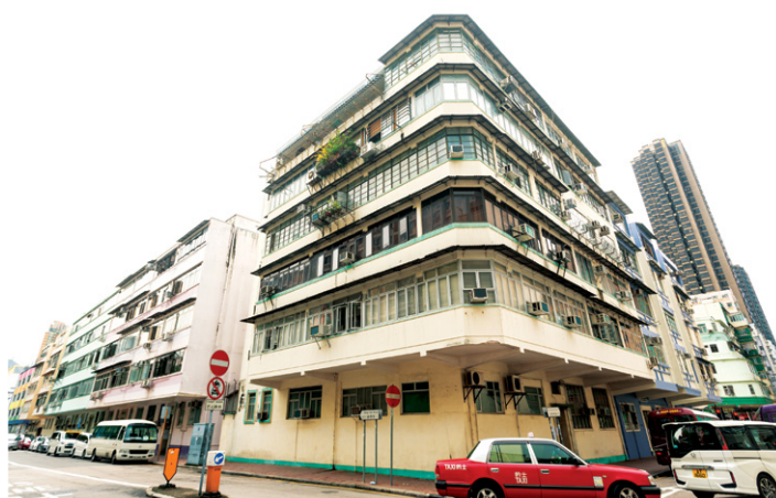
Existing view of Shing Tak Street/Ma Tau Chung Road Project
