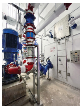
The retrofitted IB-2:SSP (left) is now equipped with new fire services systems including the Automatic Fire Alarm System (right), the Sprinkler System and tank (middle).
