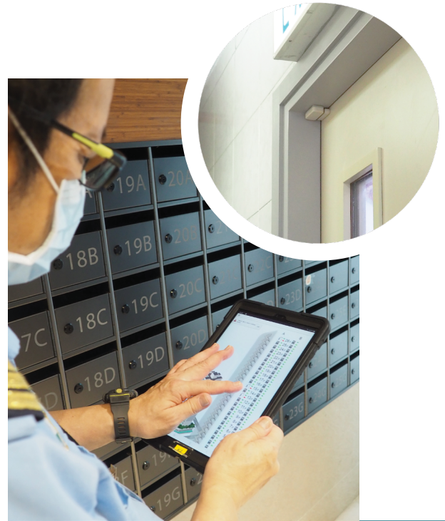
Digital remote monitoring units installed at URA's rehousing block
