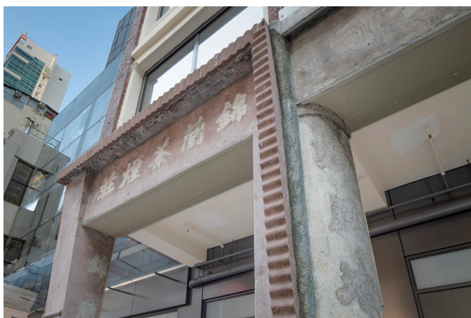
(上圖) 工人小心翼翼地將石柱的批盪逐層鑿開。 (Above) The worker discreetly removes signboard plaster on each column layer by layer.
