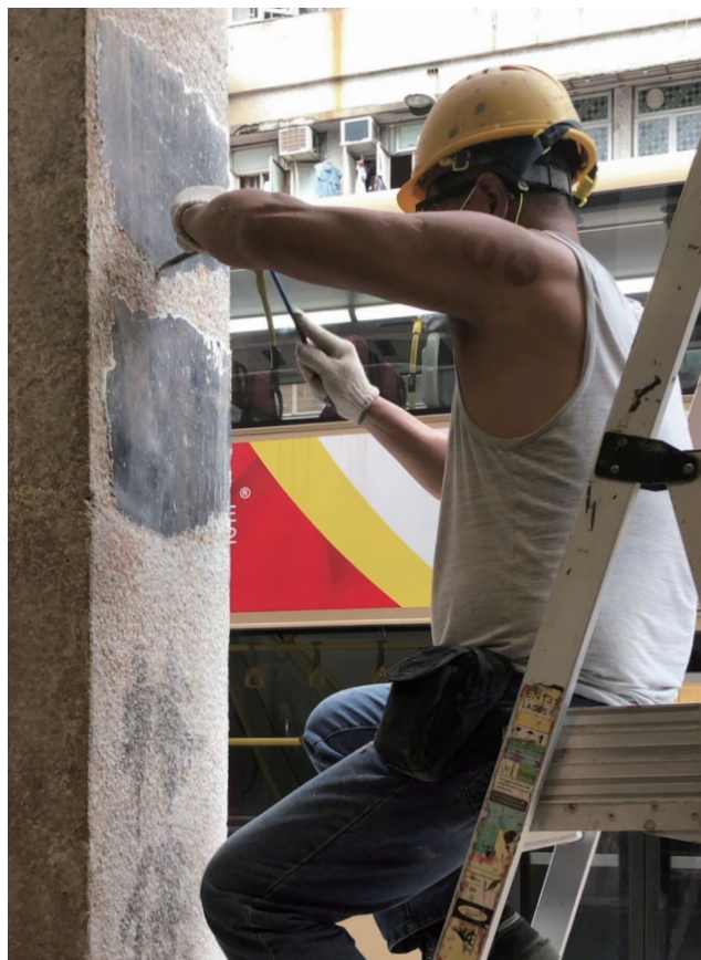
(上圖) 工人小心翼翼地將石柱的批盪逐層鑿開。 (Above) The worker discreetly removes signboard plaster on each column layer by layer.
