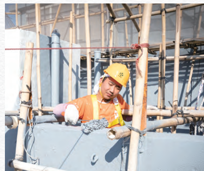
Smart Tender helps building owners procure consultants and contractors to carry out rehabilitation works.
