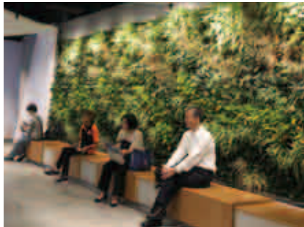
The biofilter system installed as a green wall at H6 CONET improves indoor air quality.
