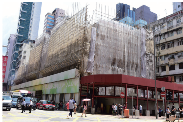
Superstructure works of Shanghai Street/Argyle Street preservation project is now in progress.
