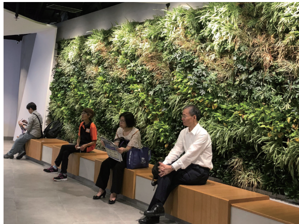
The biofilter system installed as a green wall at H6 CONET improves indoor air quality.
