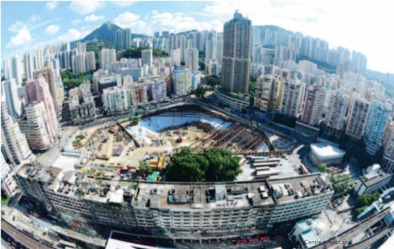
■ Panoramic overview of Kwun Tong Town Centre project site.
