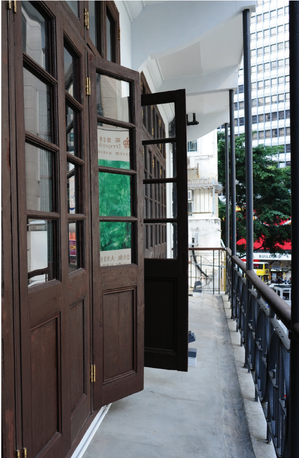
■ The project retains and preserves the character defining elements in pre-war historical buildings.
