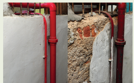
■ URA assists owners to improve building condition under IBMAS.
