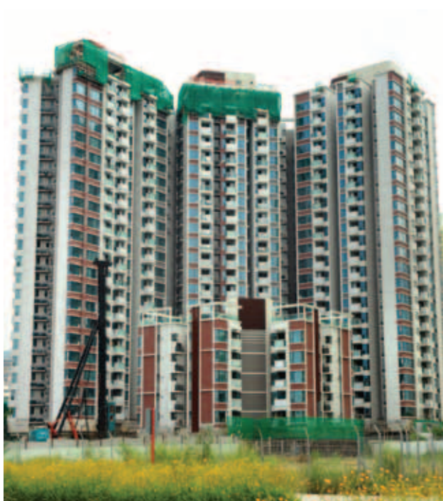
Existing view of De Novo.
