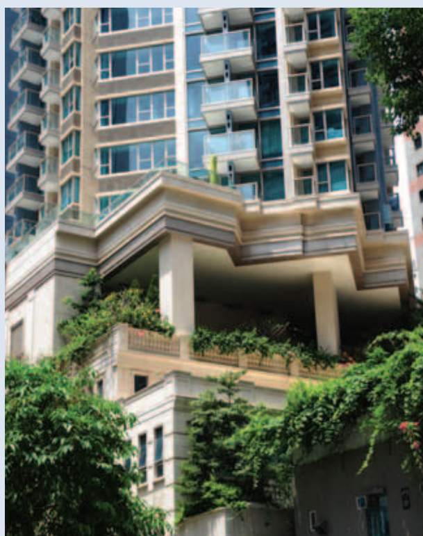
■ The construction of Lee Tung Street / McGregor Street project is nearing completion.
