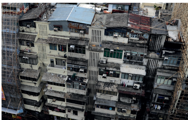
Existing view of the project.
