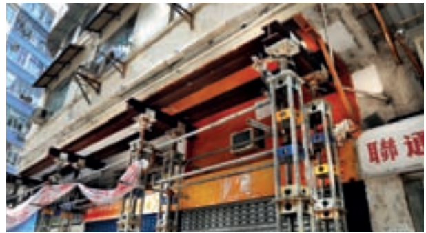
Existing site condition of Kai Ming Street Demand-led project.
