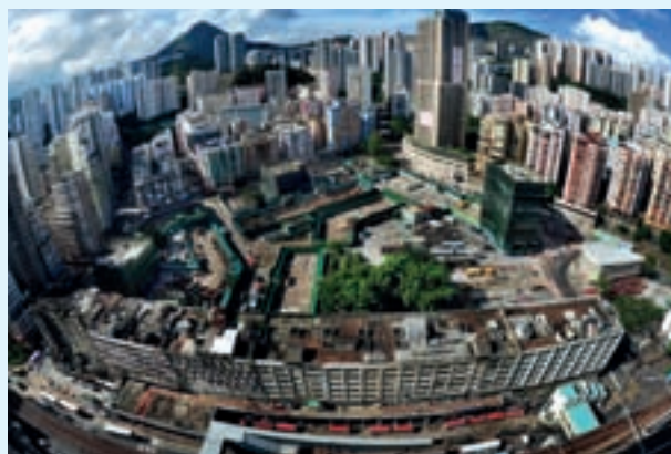
Clearance of Development Areas 2, 3 and 4 of the Kwun Tong Town Centre project is completed.
