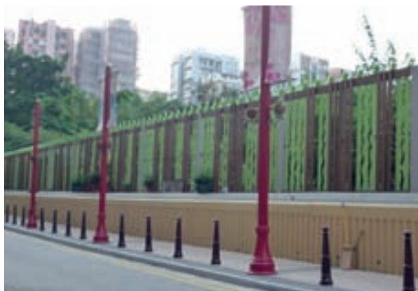
Streetscape improvement works in Mong Kok.
