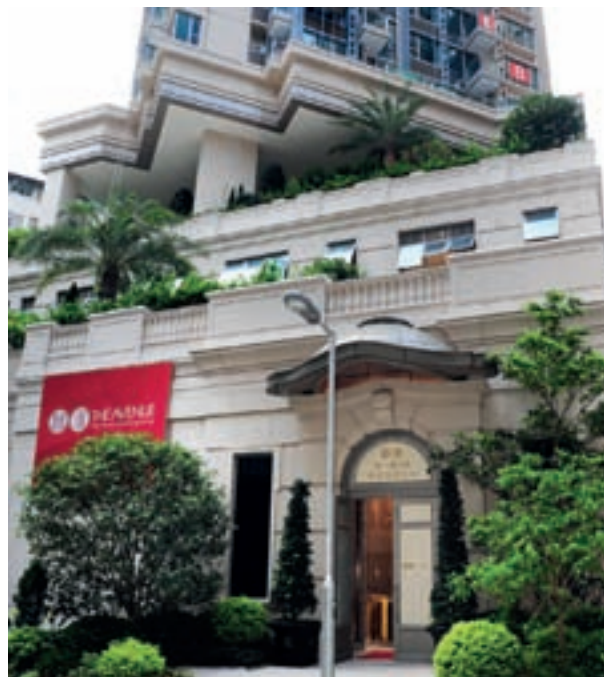
The Lee Tung Street/McGregor Street project, URA's first project to adopt environmental provisions in a comprehensive way.
