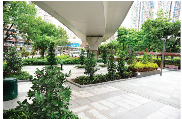
Landscape improvement work in Tai Kok Tsui.
