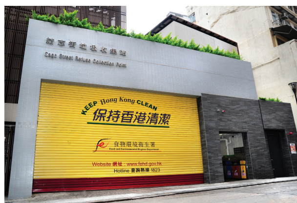
The Refuse Collection Point at Gage Street.
