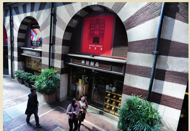
Existing view of the century old Western Market.
