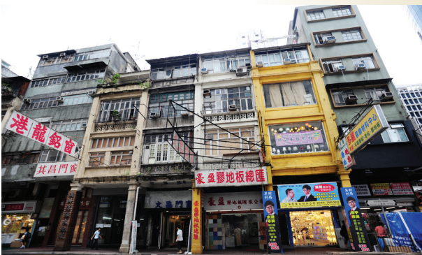
Existing view of the Shanghai Street project.
