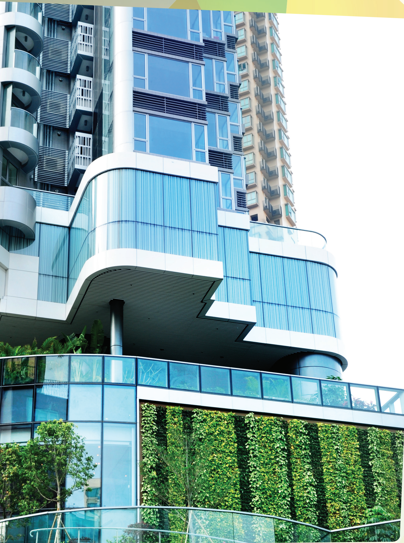
The vertical green wall featured in URA redevelopment project "One Wanchai".
