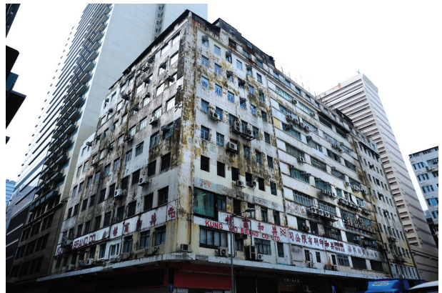
Existing view of the project.
