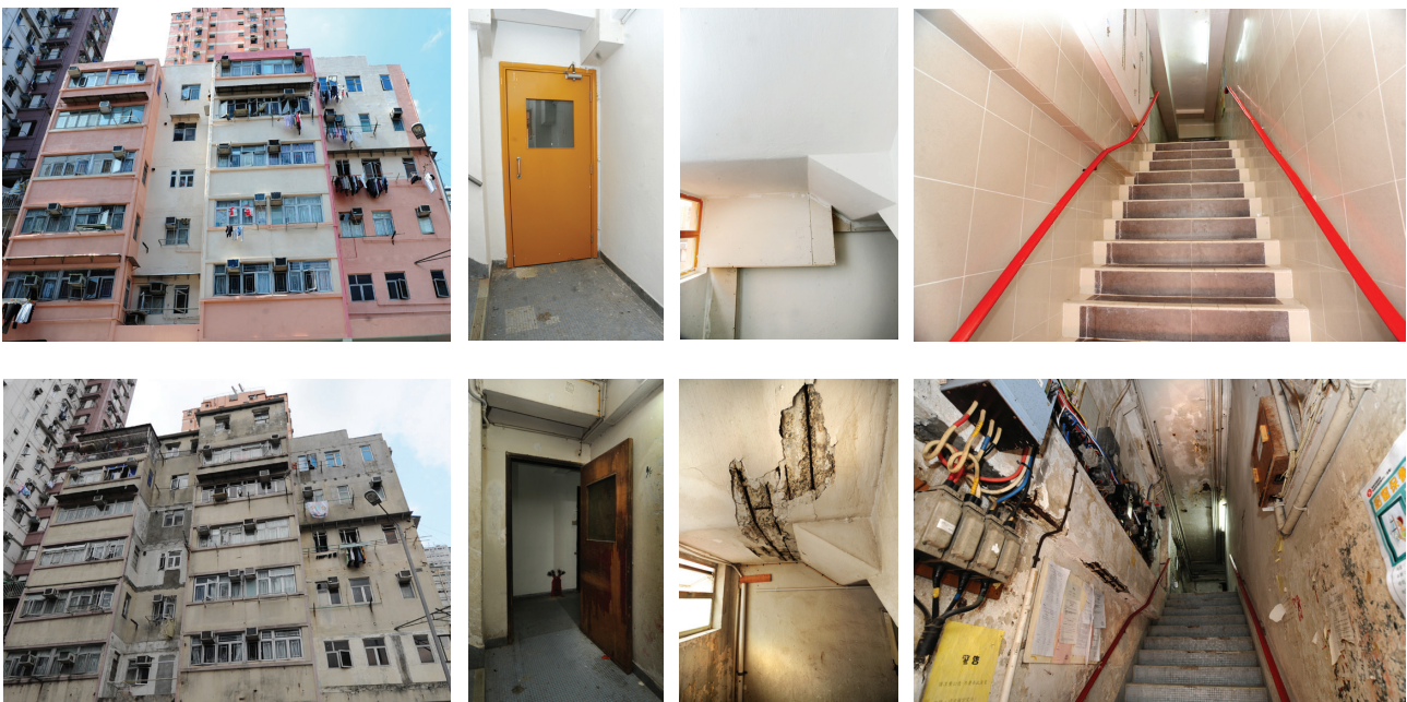
Mee Wah Building in Tsuen Wan before and after rehabilitation.
