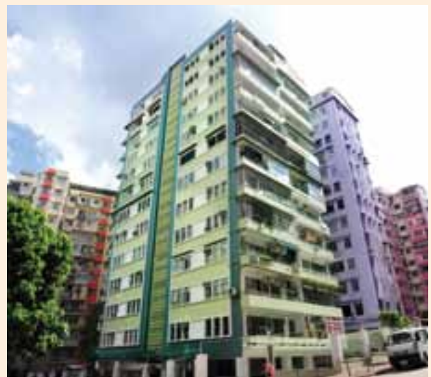
The new look of Wa Fung Mansion in Kwun Tong after rehabilitation.
