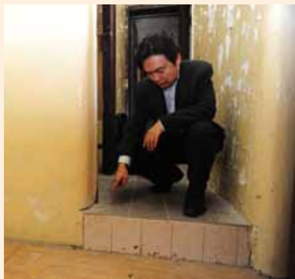
Inspection of building condition by URA staff.
