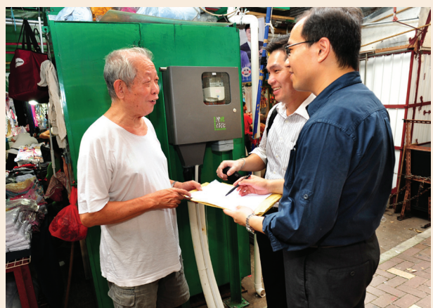
URA staff explains to a hawker about the installation of metered electricity supply.
