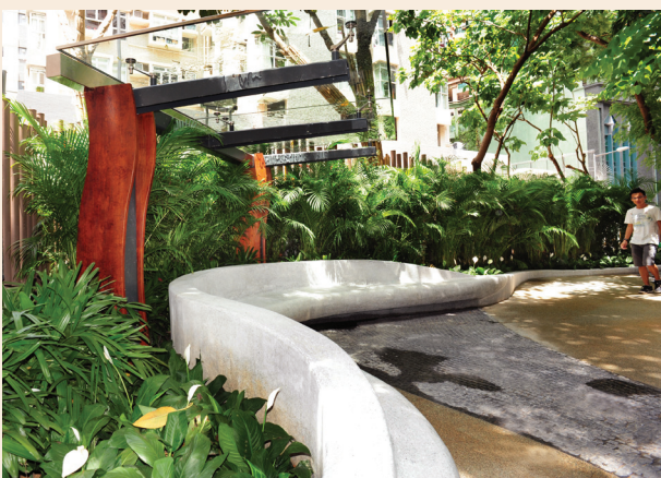
Improvement work of the open space in St. Francis Street, Wan Chai.
