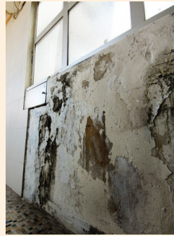
Tsui Yuen Mansion in Yau Ma Tei before and after rehabilitation.
