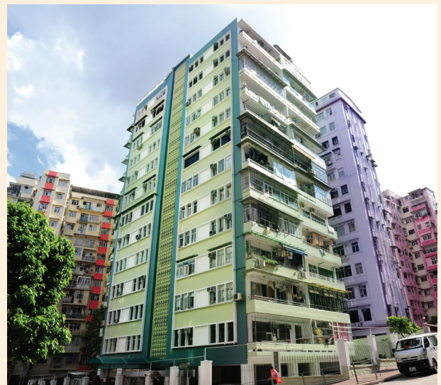
The new look of Wa Fung Mansion in Kwun Tong after rehabilitation.
