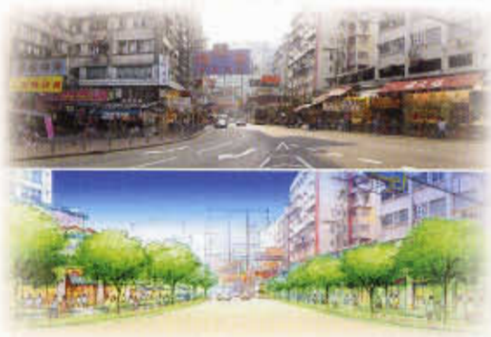
整體建築後移，令物華街擴闊33呎，再加以綠化。 Mur Wah Street will see a facelift with a 33-foot setback of building lines and widening and street-side planting.
