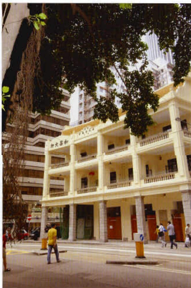
莊士敦道項目內的一列四幢廣州「騎樓式」唐樓，經翻新後的外貌。 A row of four-storey Cantonese-style terraced houses at Johnston Road redevelopment site after being preserved and refurbished.
