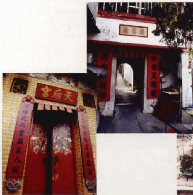
項目內三項保留的文物：天后廟、門樓及門樓上的石匾。 Three preserved items at Nga Tsin Wai Village: Tin Hau Temple, gate house and stone tablet above the gate.
