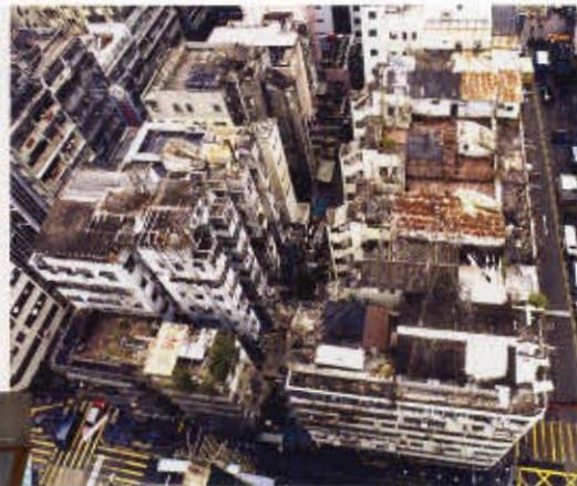
洗衣街項目鳥瞰圖。 Aerial view of the Sai Yee Street project.
