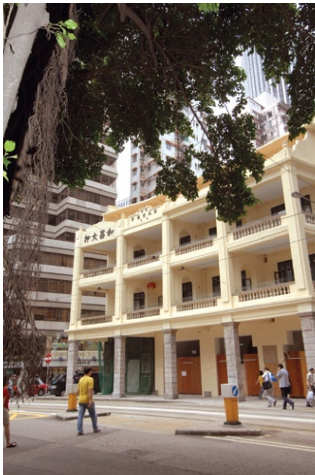
莊士敦道項目內的一列四幢廣州「騎樓式」唐樓，經翻新後的外貌。 A row of four-storey Cantonese-style terraced houses at Johnston Road redevelopment site after being preserved and refurbished.
