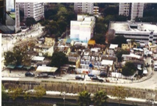
目前衙前圍村的破落狀況。 Current dilapidated condition of Nga Tsin Wai Village.
