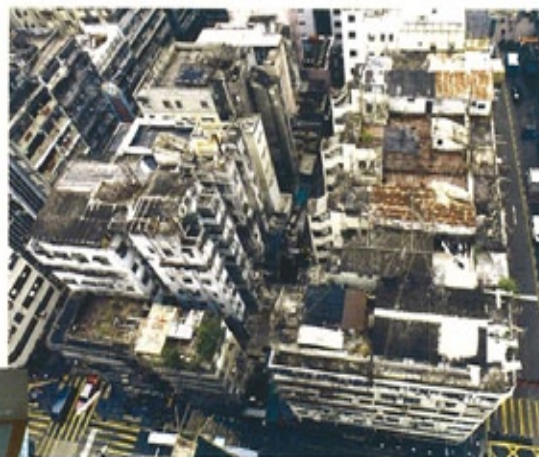
洗衣街項目鳥瞰圖。 Aerial view of the Sai Yee Street project.
