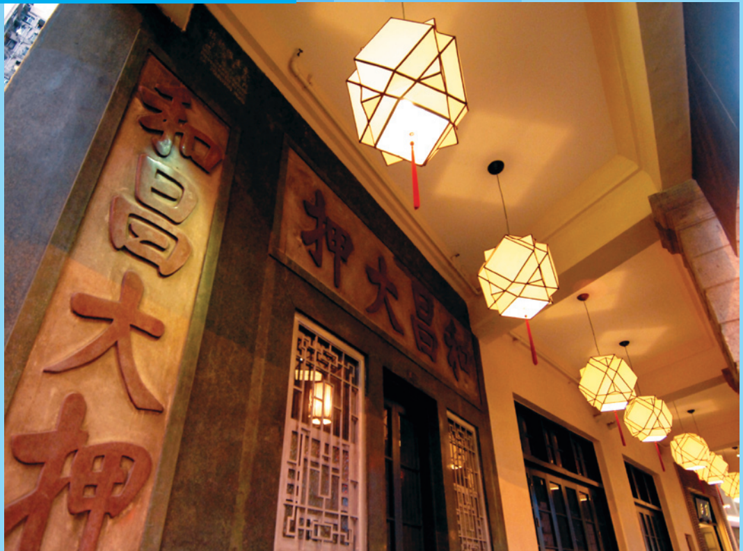
A row of four Cantonese verandah shophouses including the Wo Cheong Pawn Shop has been revitalised for adaptive re-use.
