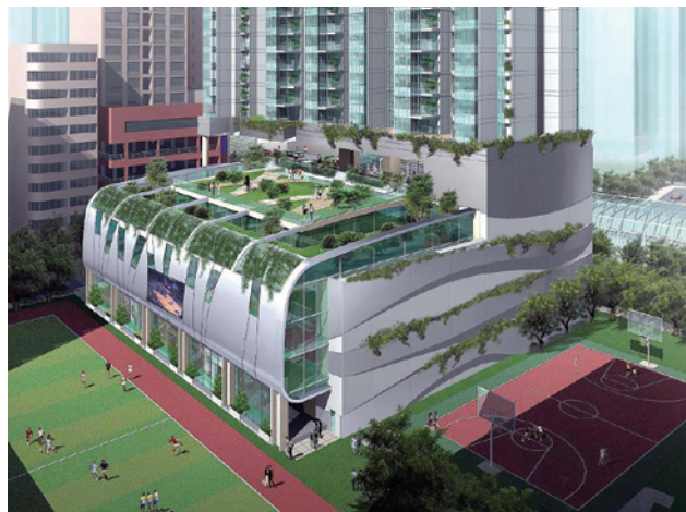
The Macpherson Indoor Stadium project delivers modern stadium facilities and a youth centre.
