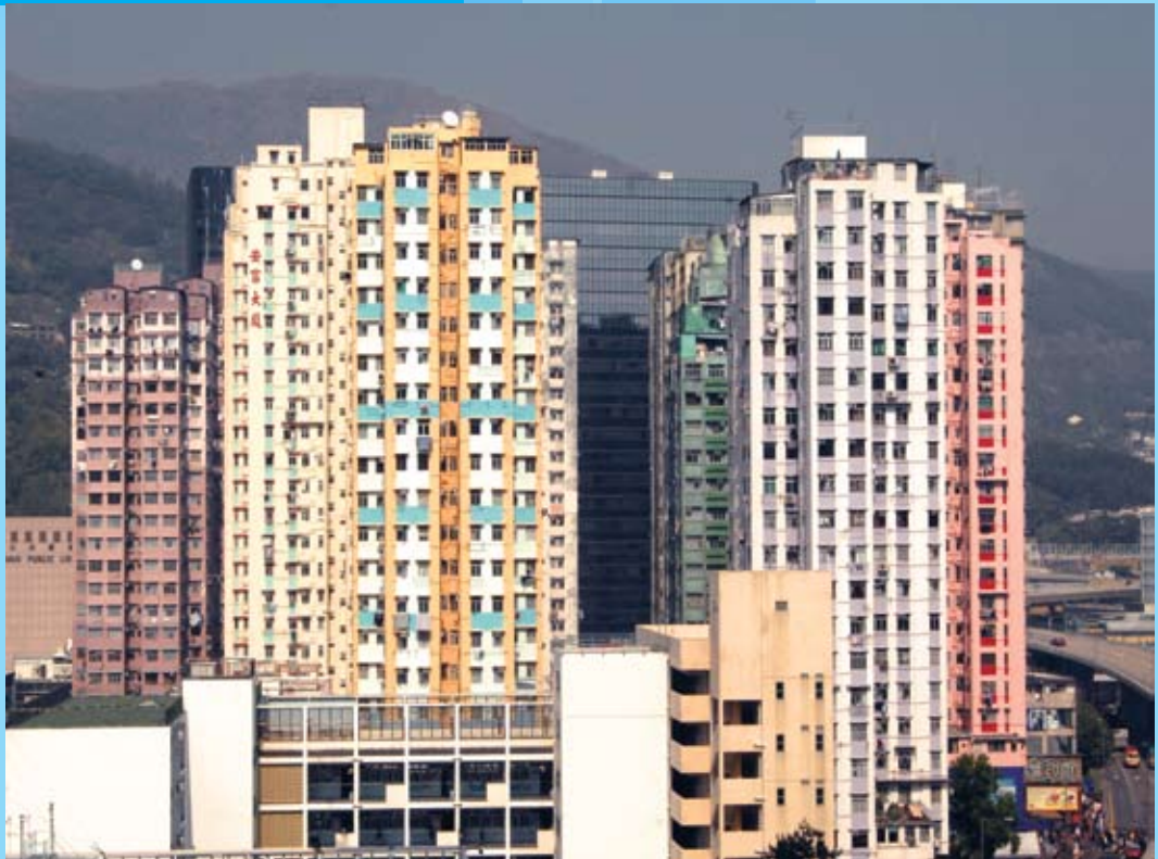
Rehabilitated buildings with thematic colour designs in Tsuen Wan.
