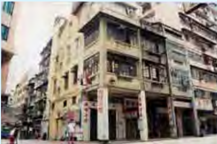
Three Cantonese verandah shophouses will be conserved for adaptive re-use.
