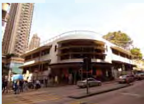
The Wan Chai Market Building (present)
