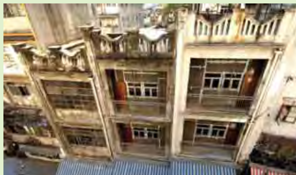
Three pre-war buildings in Graham Street will be preserved and put into adaptive re-use.
