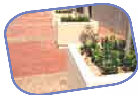
New paving and street greening in Cherry Street, Tai Kok Tsui.
