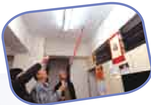
A staff member of the URA shows to a Kwun Tong resident, Mr Chu, the renovated ceiling in his flat.
