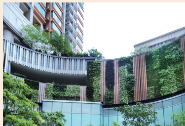
Tsuen Wan Town Centre project
