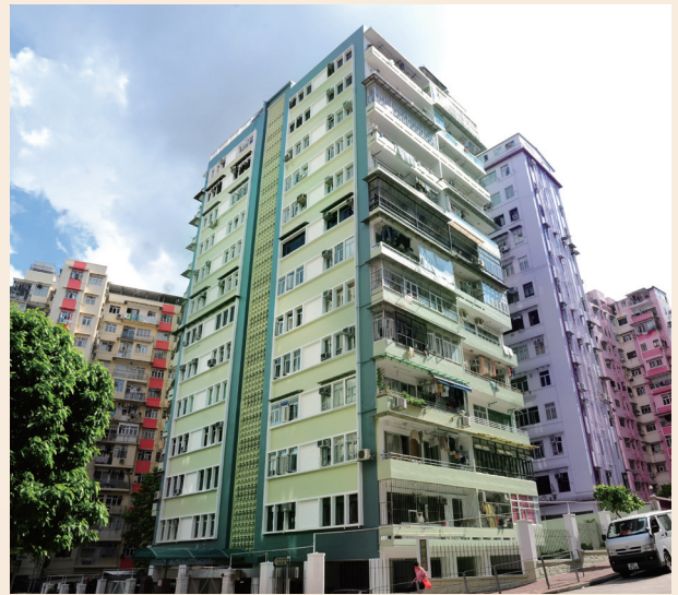
Wa Fung Mansion in Kwun Tong after rehabilitation.
