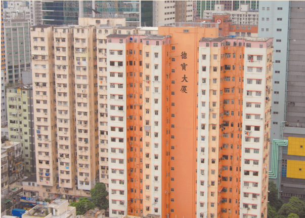
Tak Po Building in Tsuen Wan after rehabilitation.
