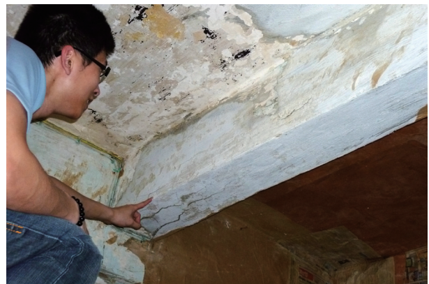
Inspection of a building's condition.
