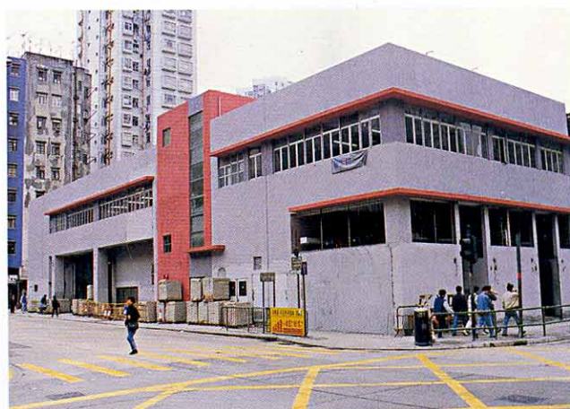
公司興建了這座臨時社區設施大樓，於一九九八年五月移交政府，使區內原有的社會福利及市政服務於重建期間得以維持。 To continue providing the existing Social Welfare and Urban Services facilities during the redevelopment, the Corporation completed this temporary GIC building and handed it to the Government in May 1998.
