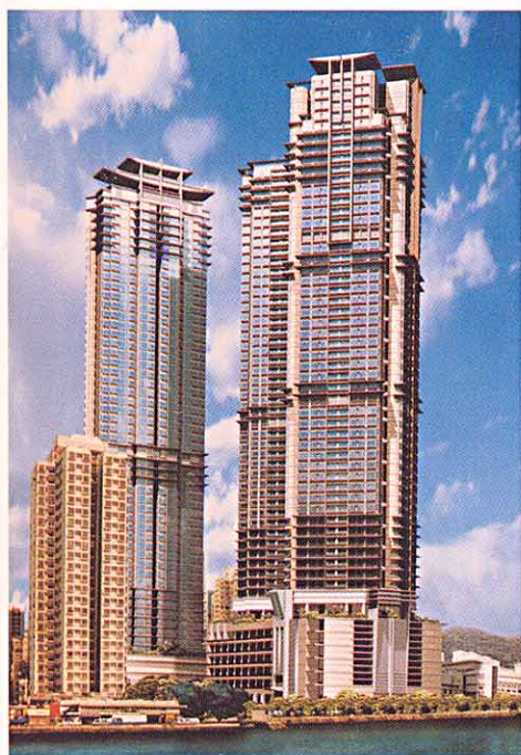
堅尼地城新海旁重建計劃未來發展外貌。 Artist's impression of the Kennedy Town New Praya redevelopment project.
