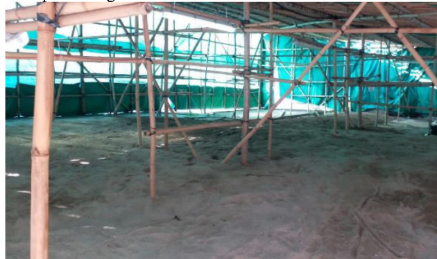
Plate 33 Last step of soil covering the sandbags
