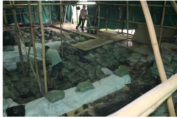
Plate 18 Stacking sandbags to the surface; looking southeast.
