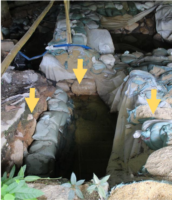
Plate 1 Split sand bags, exposed stone walls and sections not completely supported by sandbags in Trench 1
