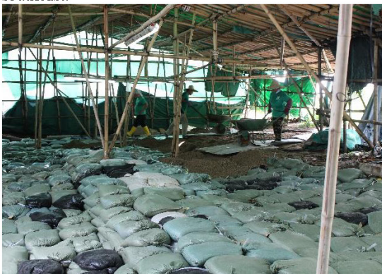
Plate 15 Adding soil to top of sandbags; looking north.
