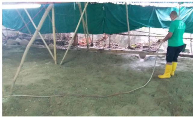
Plate 16 Water jetting topsoil, looking west.
