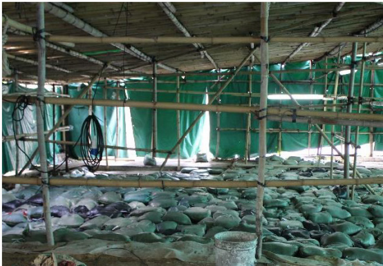
Plate 32 Surround and cover structure with sandbags
