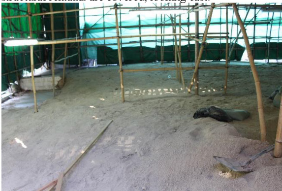
Plate 17 Adding protective geotextile to ensure all visible structural remains are covered, looking east.
