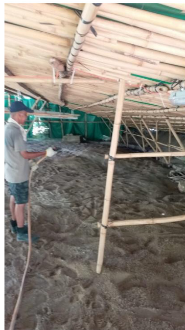
Plate 8 Water jetting topsoil, looking north.
