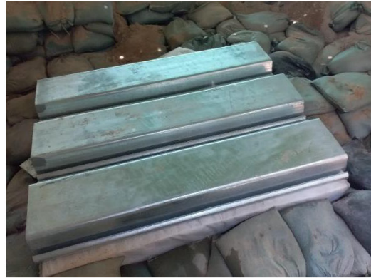
Plate 31 Adding specialized galvanized sheet piles to distribute anticipated weight
