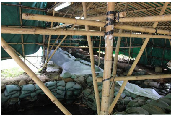
Plate 9 Adding protective geotextile to ensure all visible structural remains are covered, looking northeast.
