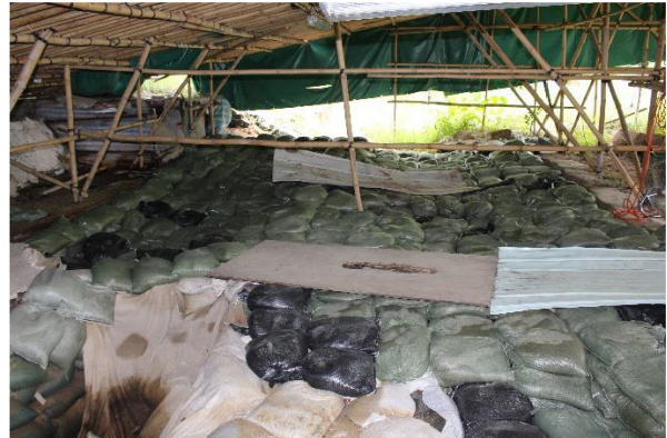
Plate 6 Stacking sandbags to the surface; looking south.
