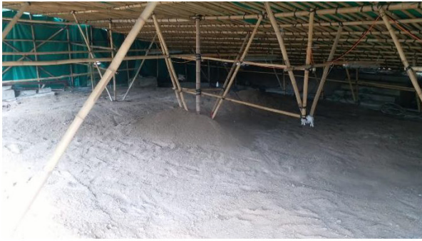
Plate 21 Backfill completed at T1, looking northeast.
