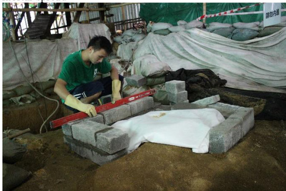
Plate 28 Building the brick wall around the stove and bonding the bricks together
