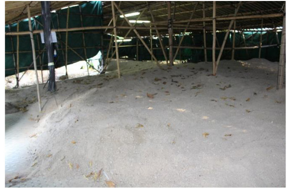
Plate 22 Backfill completed at T3, looking northeast.
