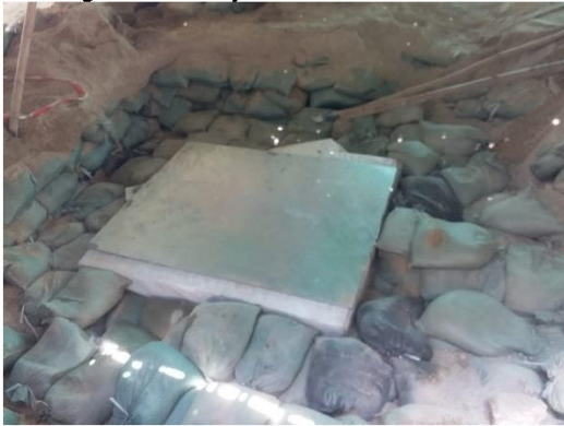
Plate 30 Adding galvanized plate to top of brick structure
