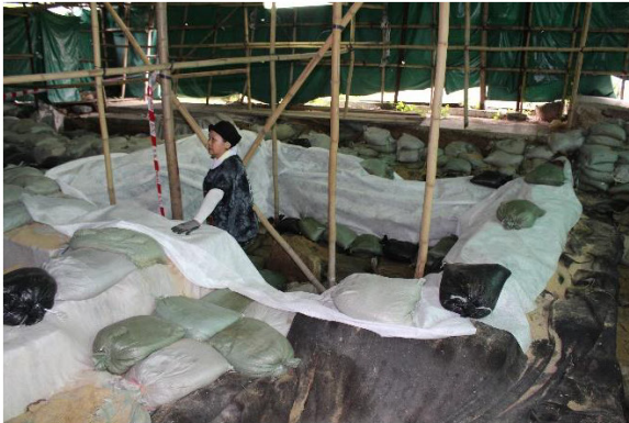
Plate 17 Adding protective geotextile to ensure all visible structural remains are covered, looking east.
