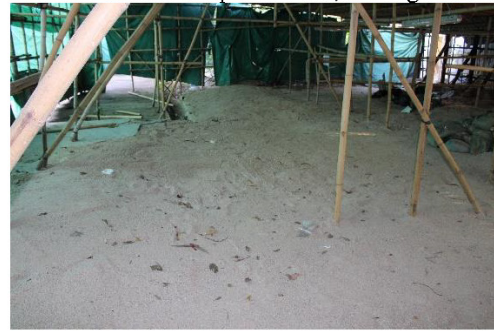
Plate 24 Backfill completed at T9, looking north.
