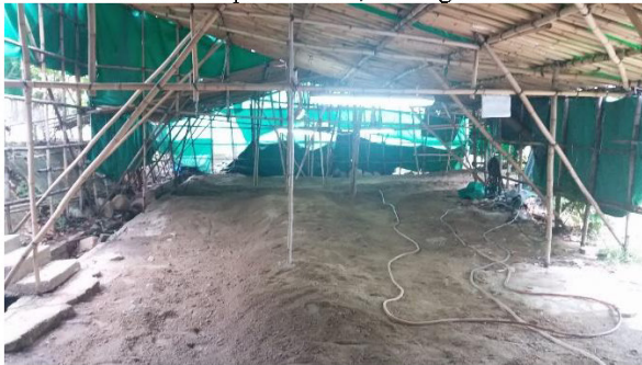
Plate 23 Backfill completed at T7, looking northeast.
