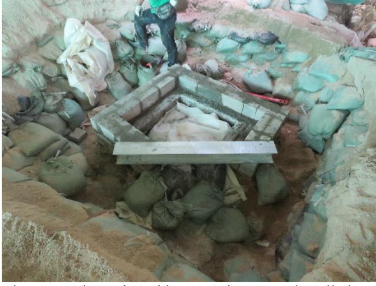
Plate 29 Universal steel beam at the corner installed to ensure greater stability.
